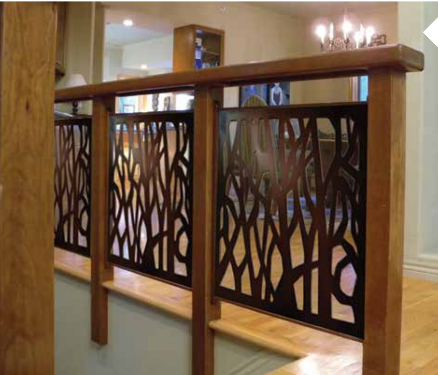
Pattern: Custom Project: Private Residence (Santa Fe, NM) Material: ¼" Aluminum Support: 36" on-center
