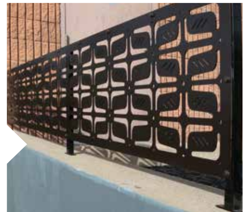
Pattern: Kenyan [ cultural ] Project: RockSol office railing (Westminster, CO) Material: 1/4" aluminum Support: 32" on-center
